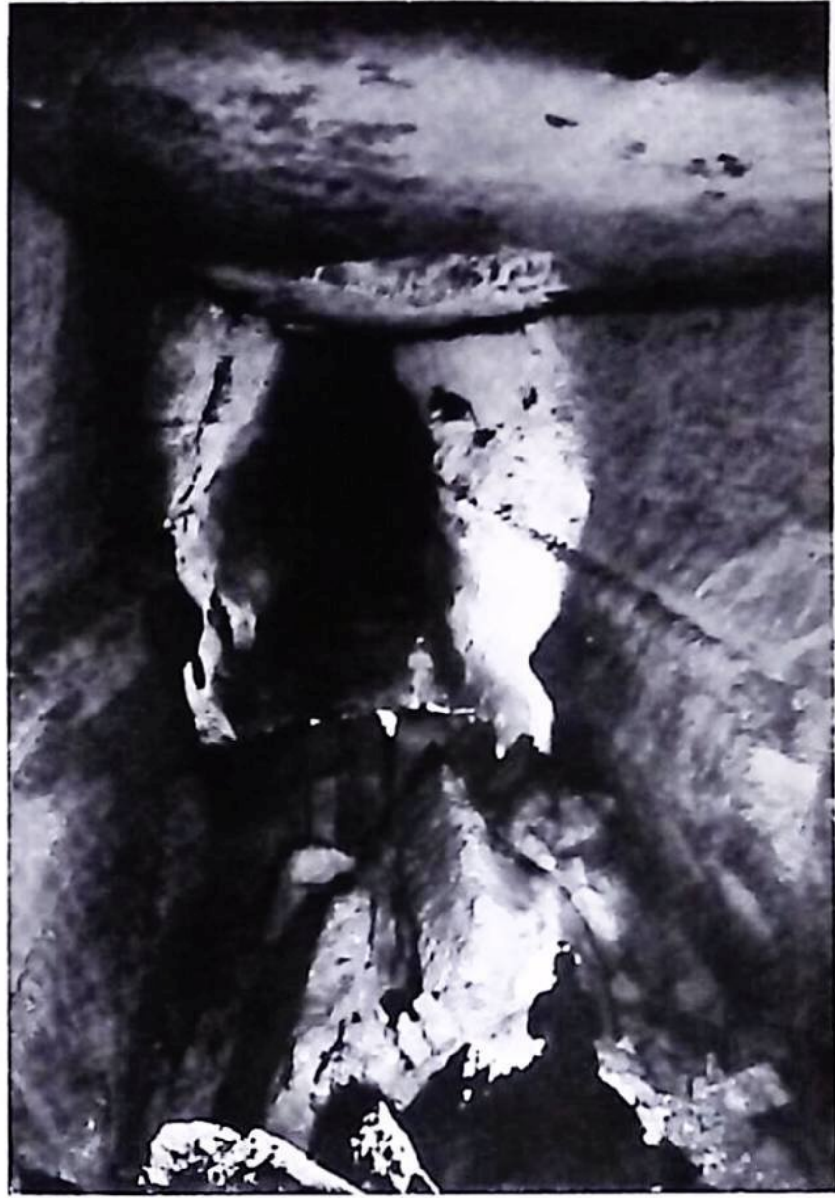
Photo 2. The main drainage outlet for Matienzo in the Llueva cave, looking upstream. The roof has been modified by collapse and the river is beneath the boulders at this point.
